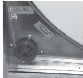
Wheel Belt & Pulley
