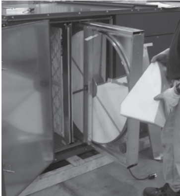
Wheel segment removed
