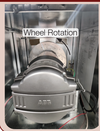
Figure 1: Supply/Exhaust Fan Rotation
